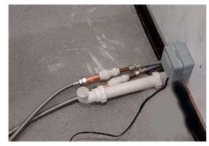
The Fuse Spur must be fitted off the floor to avoid potential water ingress should flooding occur.
